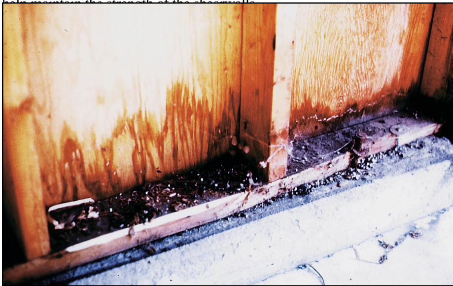
Figure 14-5 Deteriorated wood sill plate.
