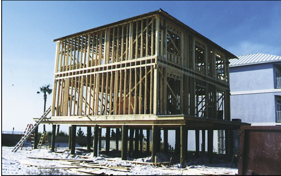
Figure 13-7 Typical wood-pile foundation.
