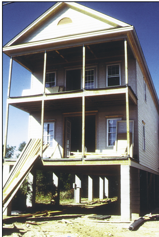
Figure 13-10 Open masonry foundation.
