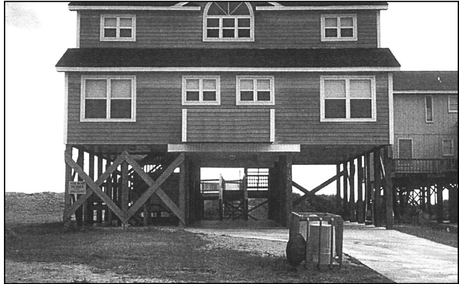
Figure 13-8 Diagonal wood bracing in a wood-pile foundation.
