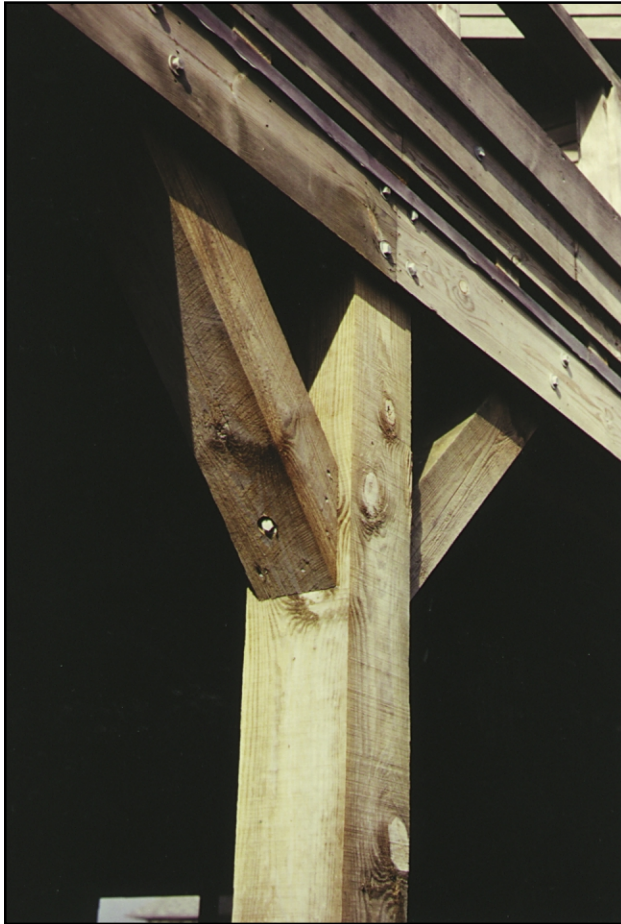
Figure 13-9 Knee bracing in a wood-pile foundation.
