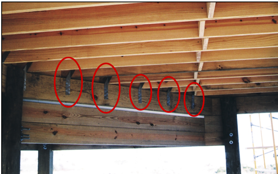
Figure 13-23 Metal twist strap ties (circled). Also, note solid blocking between floor joists.
