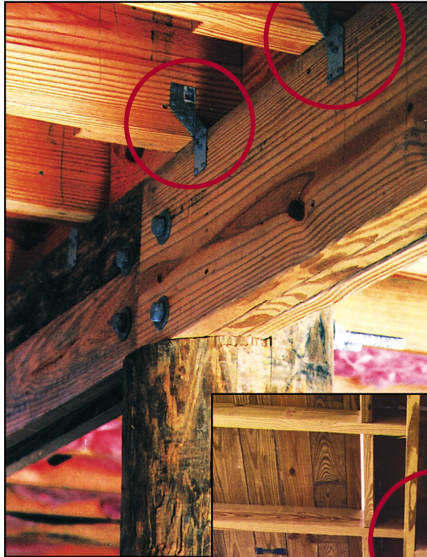
Figure 12-52 Wood joist/beam connector.
