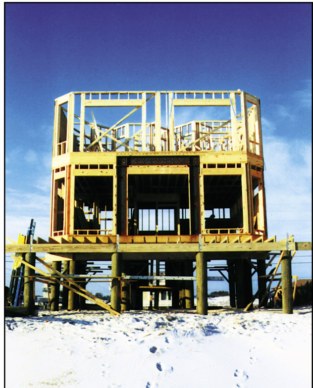
Figure 12-49 Steel moment frame at large opening.
