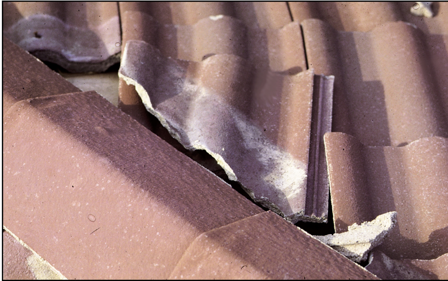
Figure 12-105 Northridge Earthquake, California. The tile in the center of this photograph slipped out from underneath the hip tiles. The tile that slipped was trimmed to fit at the hip. The trimming eliminated the nail holes and no other attachment was provided. The friction fit was inadequate to resist the seismic forces.
