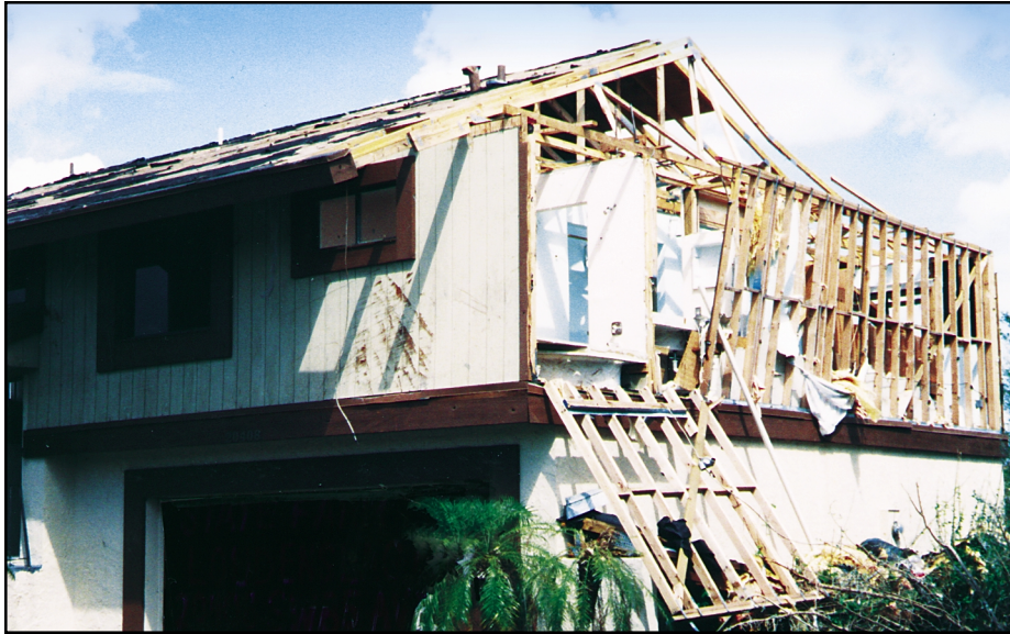
Figure 12-4 Hurricane Andrew (1992), Dade County, Florida. Second-story wood framing (on first-story masonry). End gable and wall failure.
