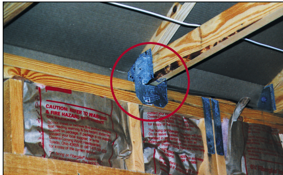
Figure 12-36 Typical connection of truss to wood wall.
