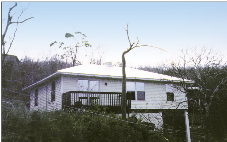
Figure 12-30 Hurricane Marilyn (1995), U.S. Virgin Islands. Hip roof that survived high winds with little to no damage.
