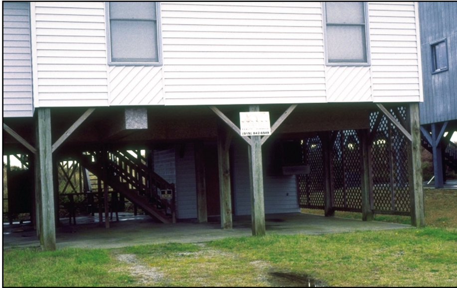
Figure 12-66 Knee bracing.
