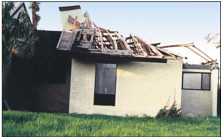
Figure 12-3 Hurricane Andrew (1992), Dade County, Florida. Roof structure failure due to inadequate bracing.
