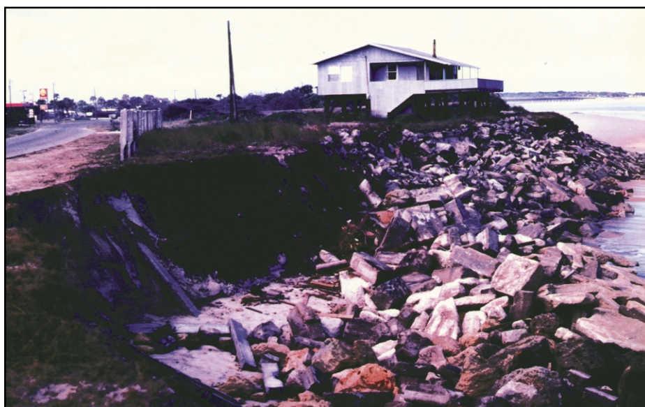
Figure 7-27 Erosion and revetment damage in St. Johns County, Florida, caused by the November 1984 northeast storm.
