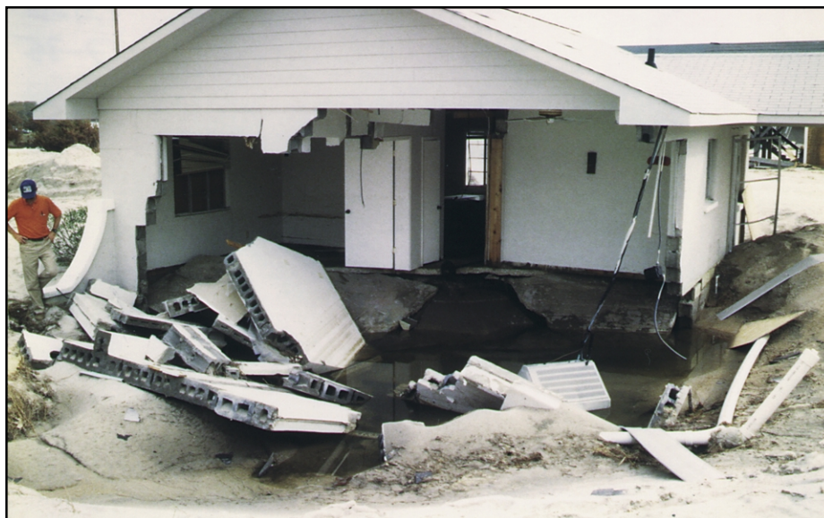
Figure 7-52 Hurricane Fran (1996). Extreme case of localized scour undermining a slab- on-grade house on Topsail Island, North Carolina. The lot was several hundred feet from the shoreline and mapped as an A zone on the FIRM prior to the storm. This case provides one argument for the treatment of these areas as coastal A zones.
