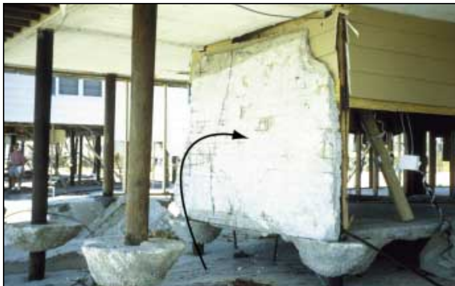
Figure 7-16 Hurricane Fran (1996). Concrete slab-on-grade flipped up by wave action came to rest against two foundation members, generating large unanticipated loads on the foundation.
