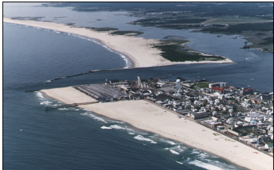
Figure 7-45 Ocean City Inlet, Maryland, was opened by a hurricane in 1933 and stabilized by jetties in 1934-35. Note extreme shoreline offset and downdrift erosion resulting from inlet stabilization. 1992 photograph.
